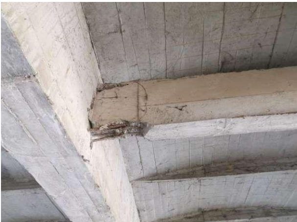
图 2-27 1-7#横系梁剥落露筋
